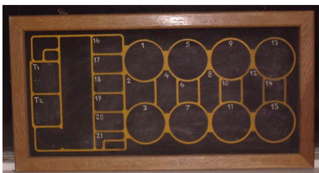
Figure 1. Chalk board of the kind that used to be in all control rooms. It represents the different silos and was used for marking the kind of grain stored in each silo.
